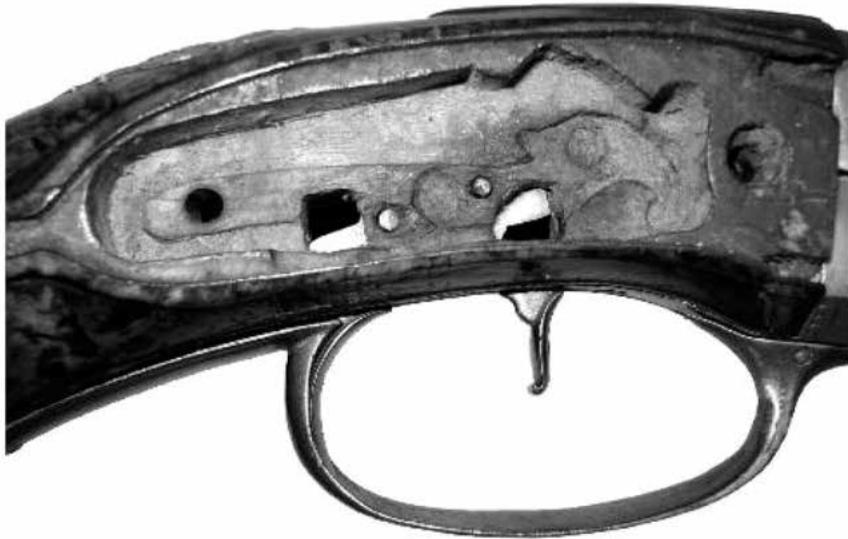
Fig 4. Stock cut out for right lock. Forward trigger serves top barrel by pushing down on sear of right lock while rear trigger pushes up on sear of left lock to fire lower barrel.
