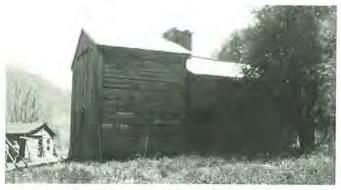
Figure 6b: The back of the Shell homestead as it appeared in 1975 clearly shows the earlier, taller cabin on the left, and the later, lower addition on the right. Both sections have an upper or second floor. Note the original clapboard siding high up under the eves on the end of the house, indicating that the entire house was sided at one time, but over the years the siding was lost or removed. Courtesy Kentucky Heritage Council, Frankfort, Kentucky
