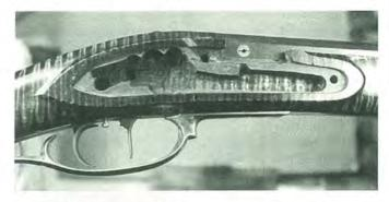
Figure 9. This lock mortise has been carefully reinforced with epoxy to resist chipping during lock removal, while still letting the grain of the mortise show through.
