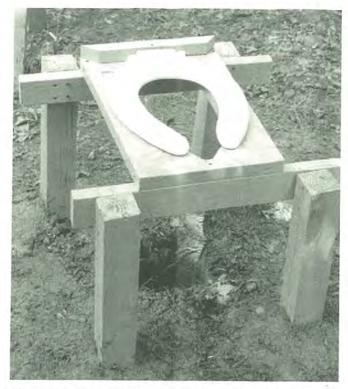
Figure 3 – The basic structure is a salvaged toilet seat on a framed support. Some codes will require the toilet structure to be framed in and vented with screened openings.
